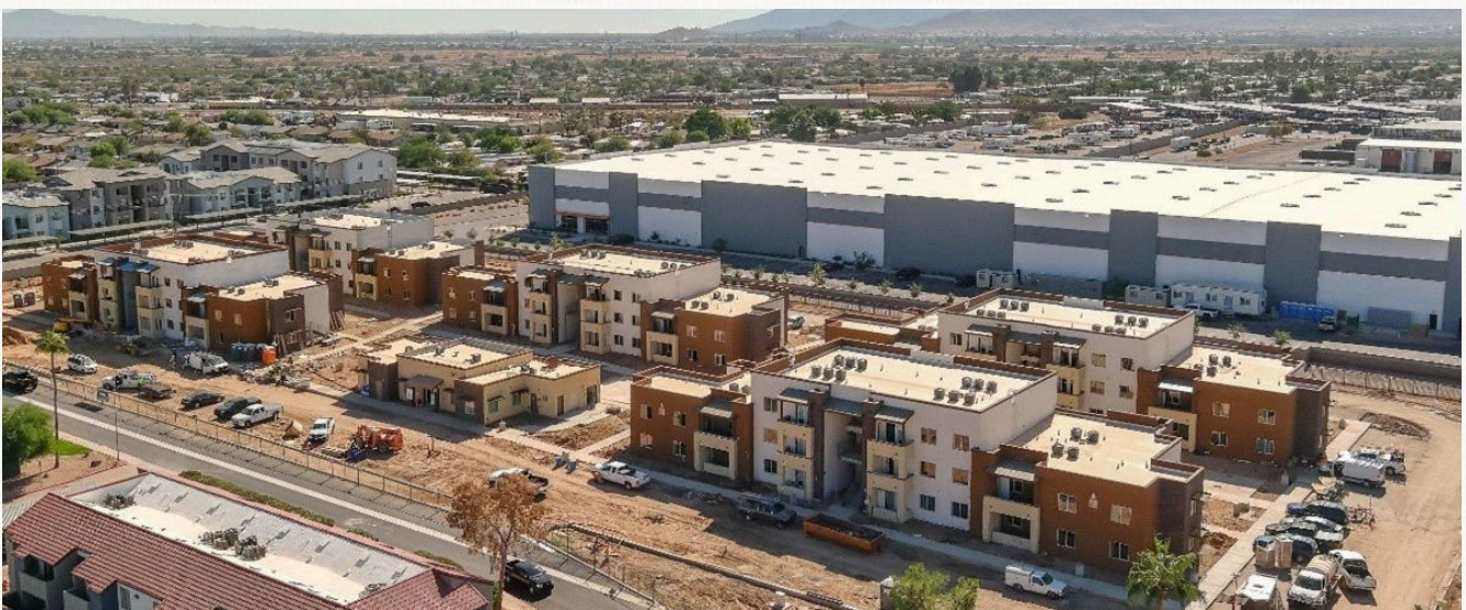
Norton Circle Apartments (Aerial photo during construction)
