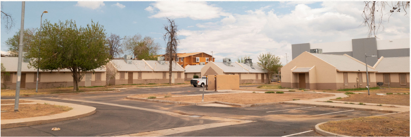
Norton Circle Apartments (Pre-construction)
